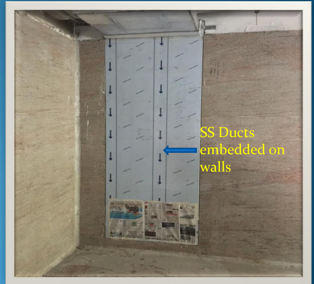
SS duct embedded in walls
