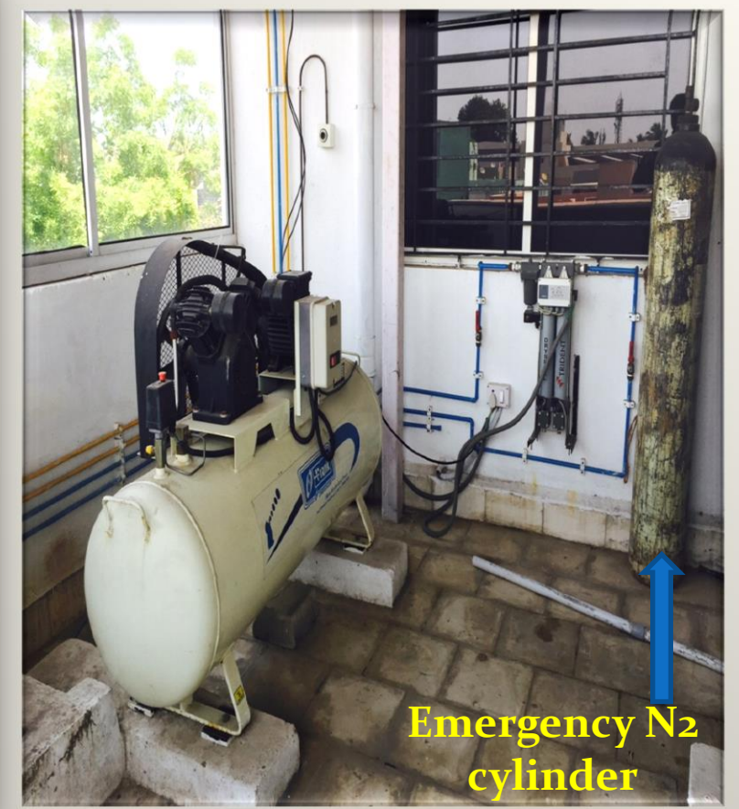
MEDICAL GAS COMPRESSOR+FILTER
